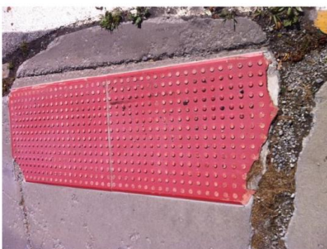
Figure 1. VTrans Plastic DWP (Installed 2004, Photo 2013)
