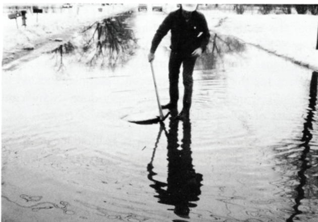
Copies of slides showing actual manhole lid inflow.
