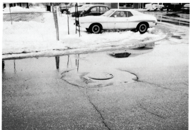
Copies of slides showing actual manhole lid inflow.
