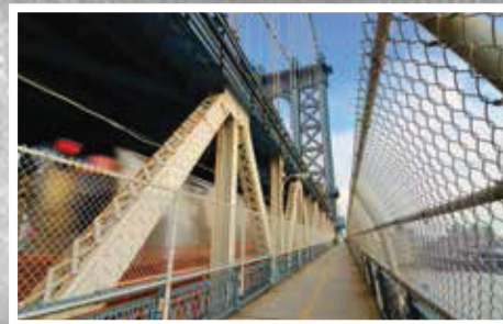
FABRICATED SAFETY FENCING
