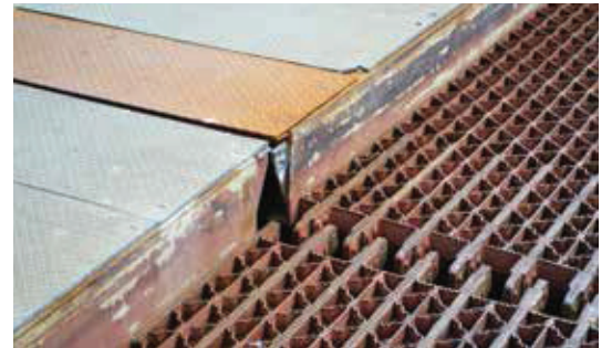
EXPANSION JOINT SECTIONS
