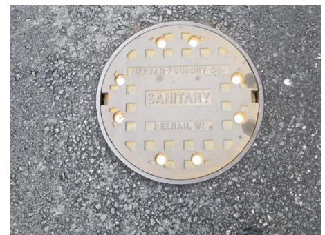
Installed 1772 manhole cover with new venting (courtesy, City of Fort Wayne, IN)
