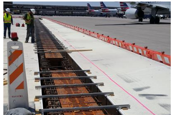
4993 Trench Formed and ready for pouring.
