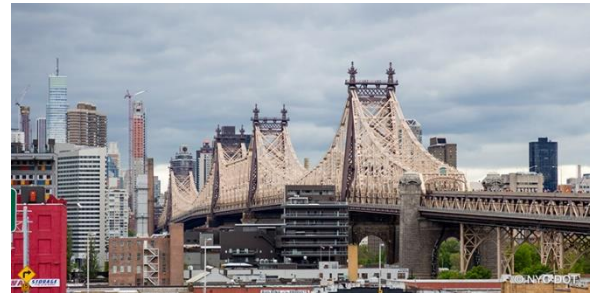
View of Ed Koch Queensboro Bridge looking towards Manhattan from Queens (Source – NYCDOT)
