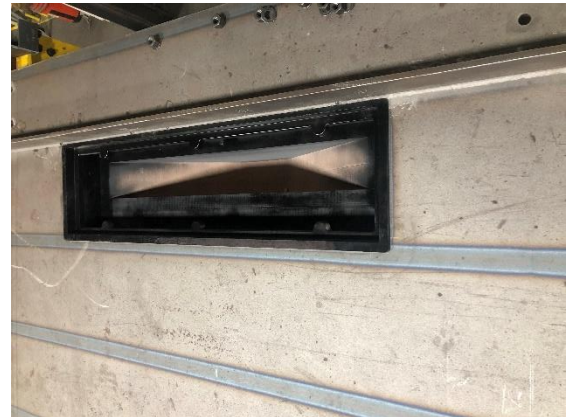
Prototype Scupper in Steel Deck
